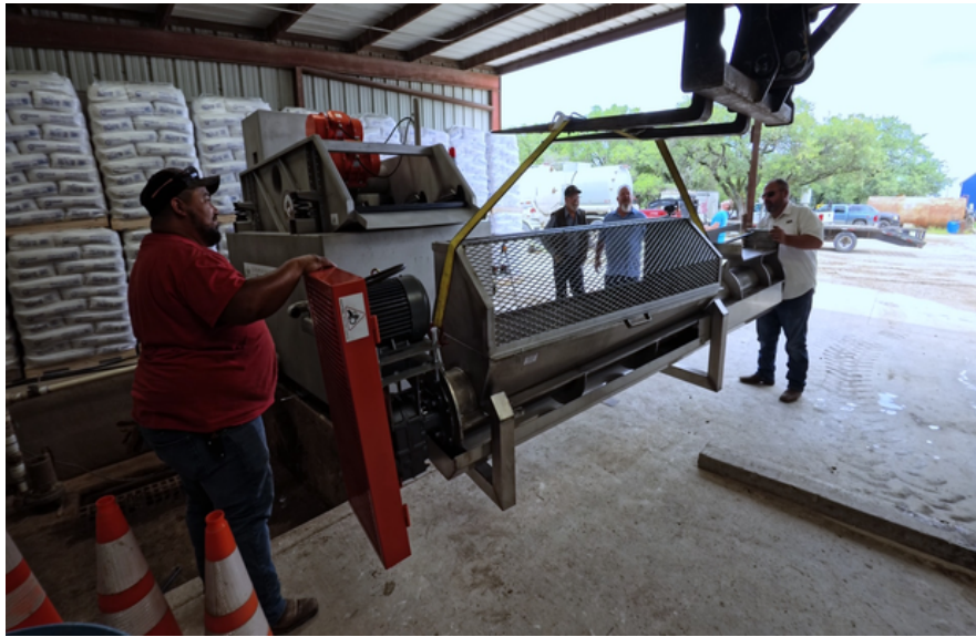
Auger assembly suspended during installation using a telehandler, shackles and lifting straps.
