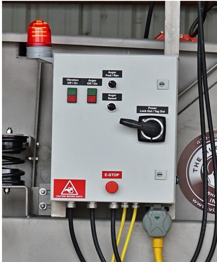
Control panel — Vibration Off/On, Auger Off/On, Auger Fwd/Rev, Auger Speed, Power Lock Out/Tag Out disconnect, and E-STOP button
