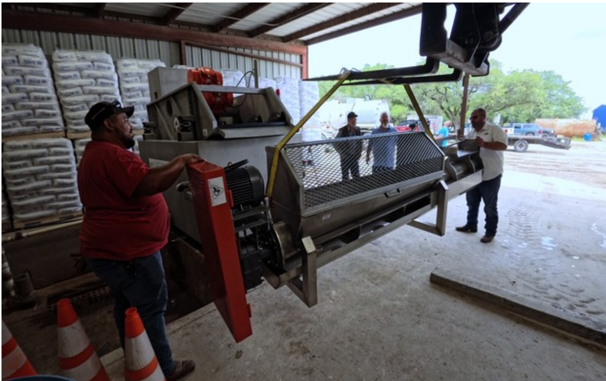
Auger assembly suspended during installation using telehandler, shackles, and lifting straps
